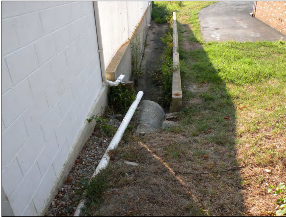
5. Outlet conduit and discharge channel.
